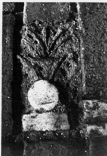
Figure 8.54. Church wall, detail.
