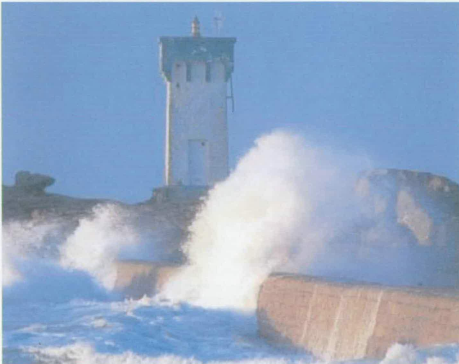
Figure 2.1 Wave overtopping at a monolithic breakwater (© Gerard Fournier / Editions Jos le Doare)
