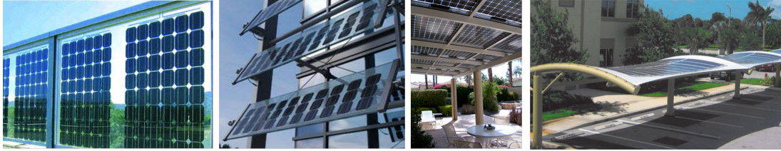
Figure 6.20: Examples of BIPV balustrades, louvres, canopies and carports (photos courtesy of Green Coast Solar, Colt, Solartec and Skyshades).
