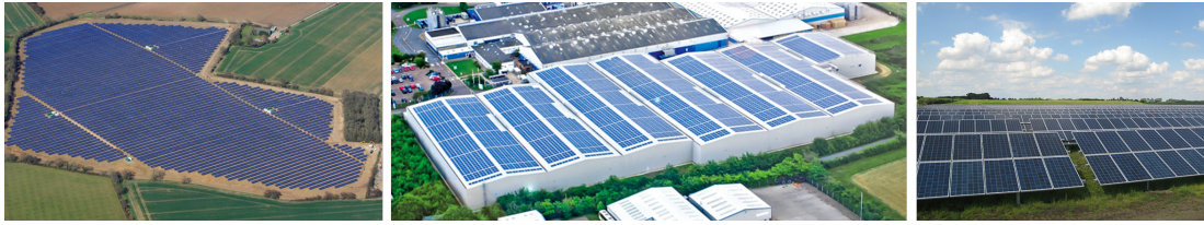
Figure 6.13: Examples of utility-scale solar projects in the UK (photos by Lightsource Renewable Energy Ltd).
