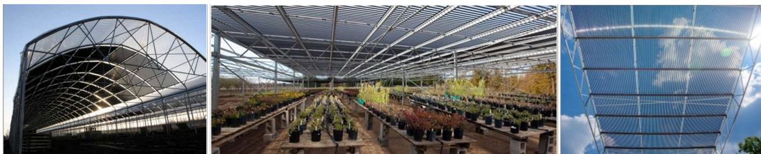
Figure 8.5: Examples of BIPV installations by Solyndra [GTM (2010-2014)].
