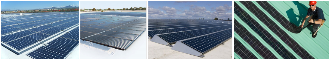
Figure 6.17: Examples of BIPV on flat roof (photos courtesy of Lumeta, Solyndra, Sunpower and Solopower).
