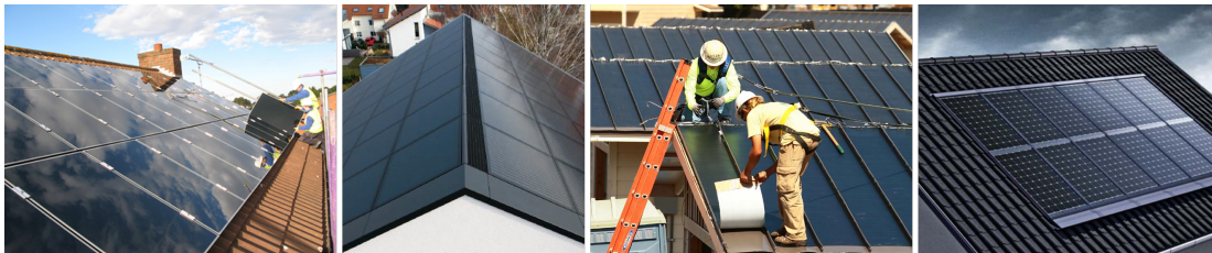
Figure 6.15: Examples of BIPV on sloped roofs (photos courtesy of Hanergy, Systaic, Unisolar and Solon).
