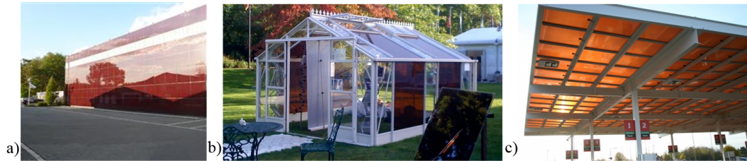
Figure 8.9: Examples of BIPV installations by Polysolar: a) facade in Dortmund, b) PV greenhouse and c) petrol station canopy in the UK [Polysolar (2014a)].
