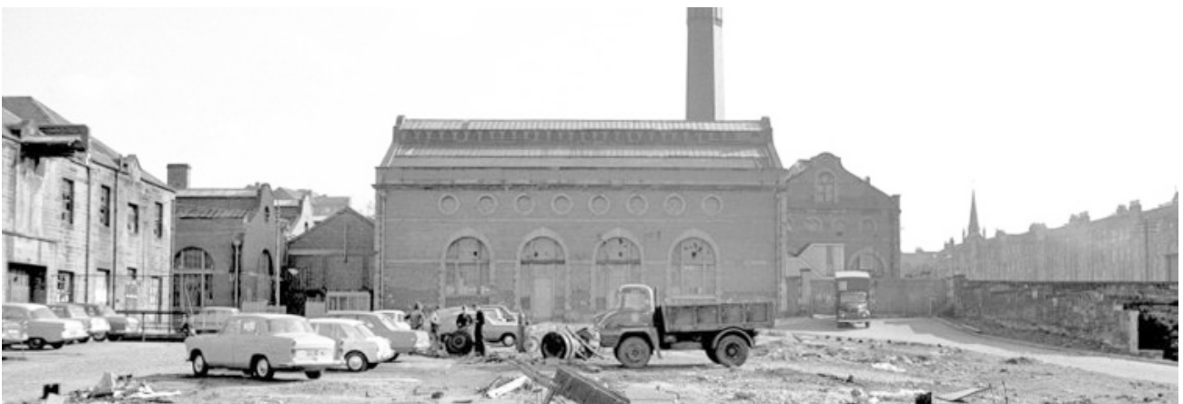
Figure 5: View of the old depot from northwest, Image from CANMORE
