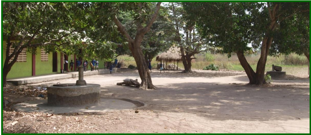
Figure 93: Missing school well hand-pumps - Mathinka Bana
