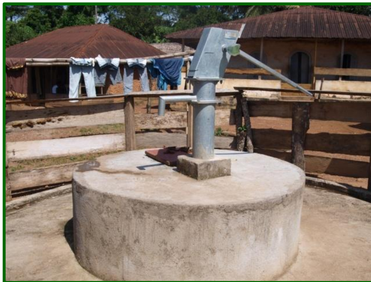
Figure 38: Example of a water point with 'no failure' - Rowunkor
