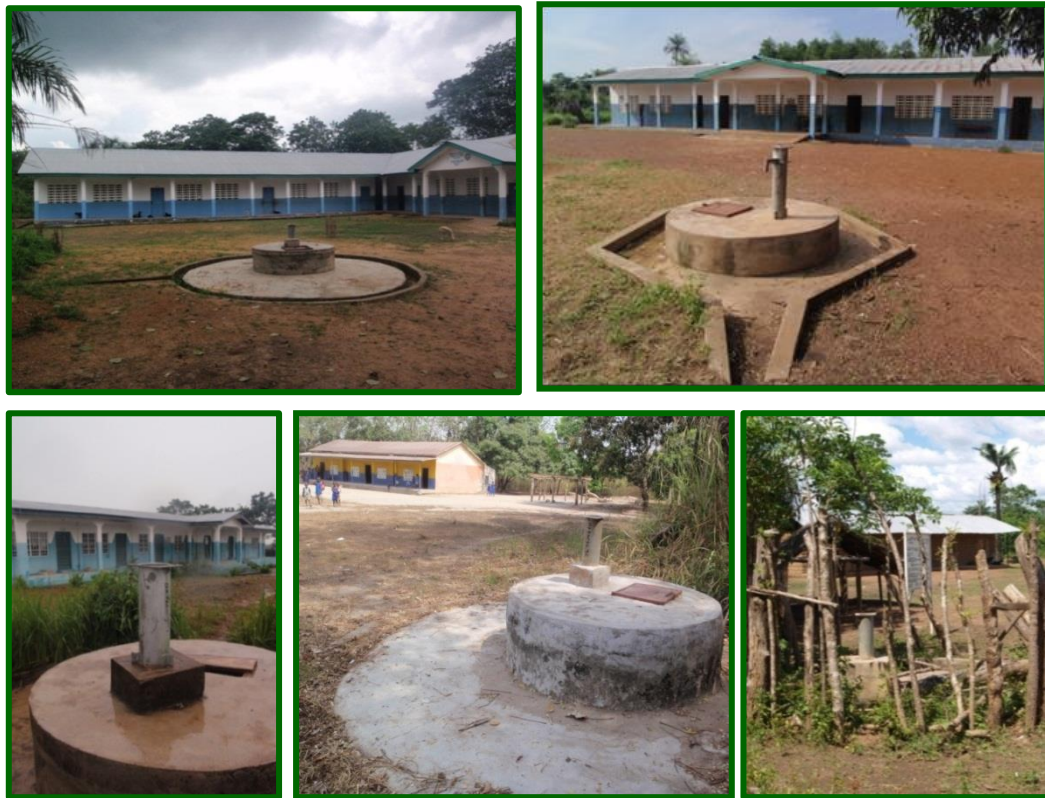
Figure 91: Compilation of various primary school wells in Tonkolili District
