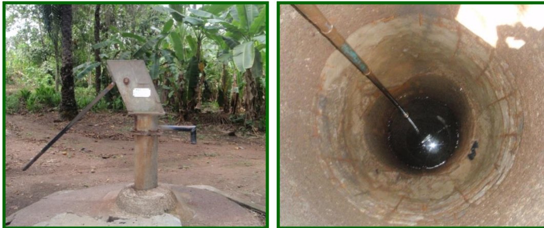
Figure 34: Example of Grade B failing - Romankro
