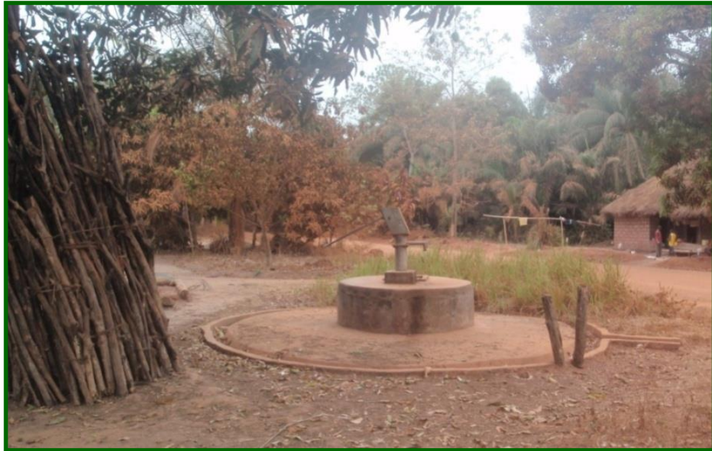
Figure 50: The missing fence - Matukutu 2
