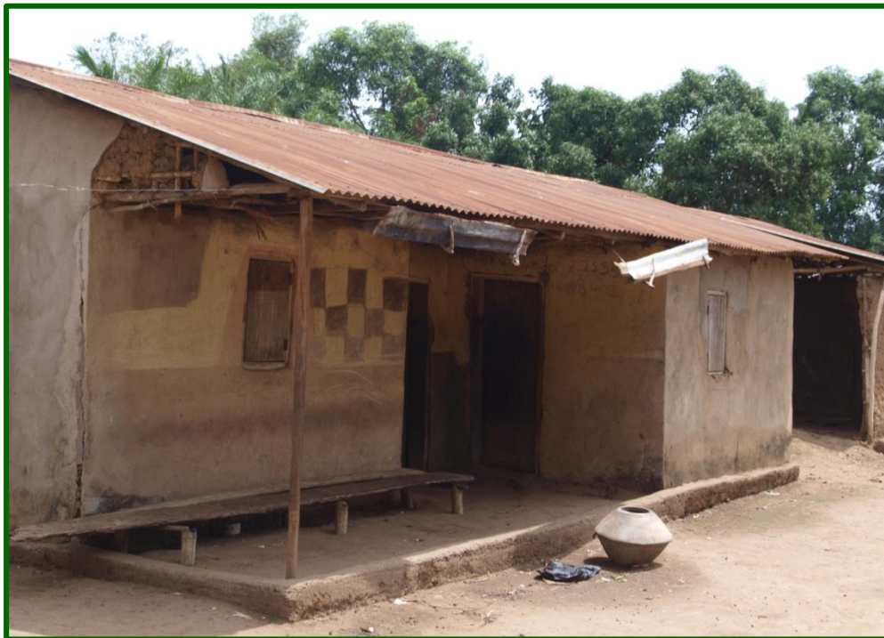
Figure 83: Example of permanent rainwater collection container - Robis
