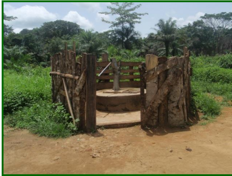
Figure 37: Example of Grade E failing - Mathombo
