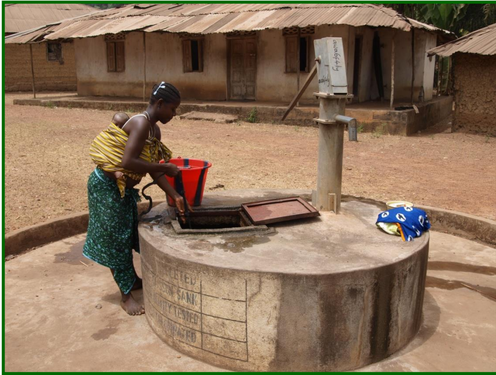
Figure 53: Example of a non-chlorinated well - Kumrabai Station
