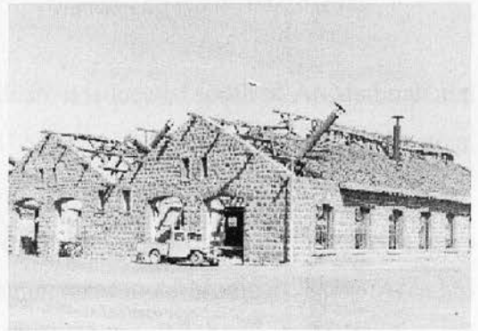
Figure 7IV.55: Railway stores building
