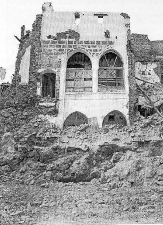
Figure 7I.3: Quarter of al-Aghwāt, the traditional courtyard house, during demolishing
