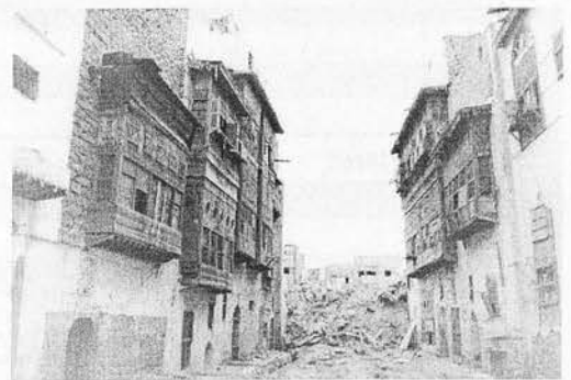
Figure 7I.4: Zuqāk al-Şulġān in al-'Anbariyah area, during demolishing
