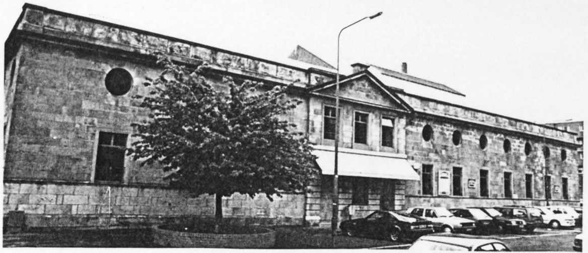
Elevation of Baths Following Refurbishment
