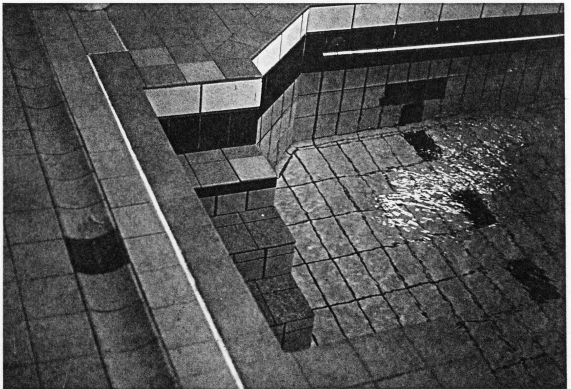
46. Stair shape retained, modern handrail reflects original fixture- Dalry, Edinburgh.
