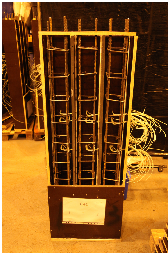
Figure 3.3: Column formwork used in casting
