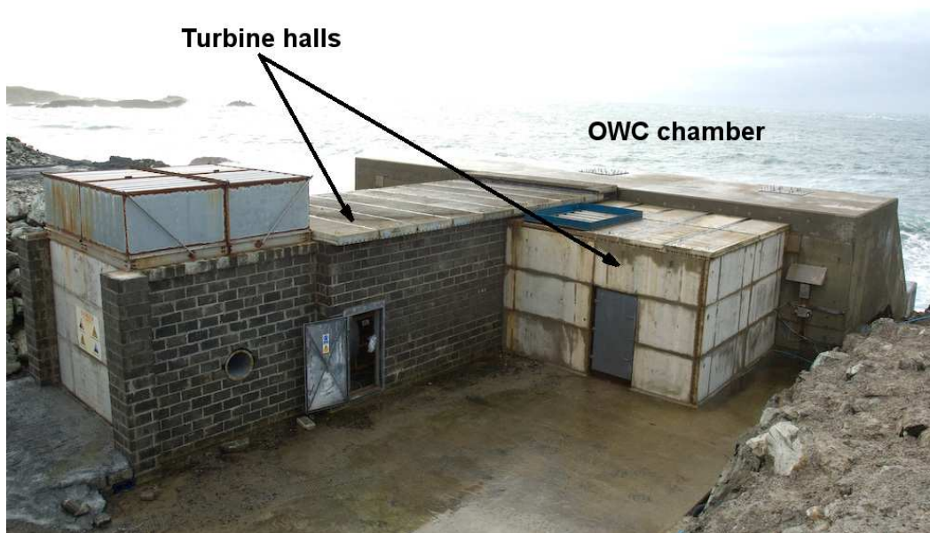
Figure 10: Turbine halls connected to OWC chamber
