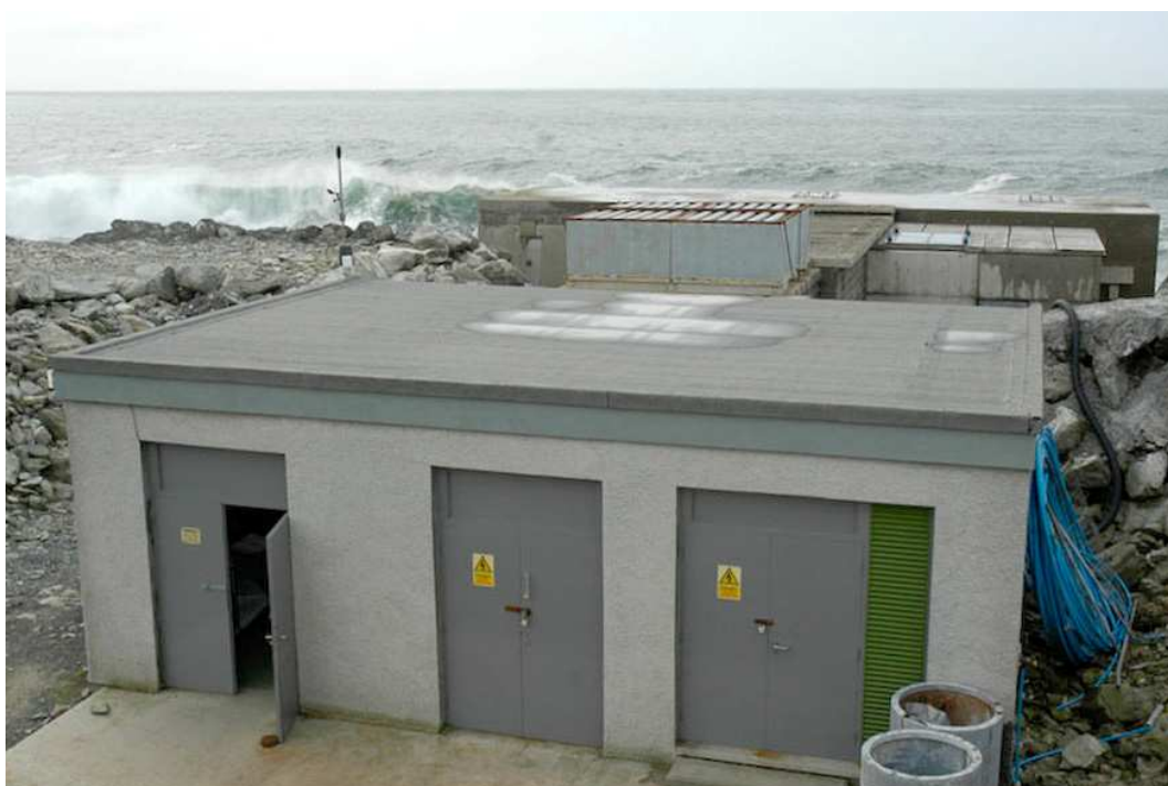
Figure 11: Control room (foreground)
