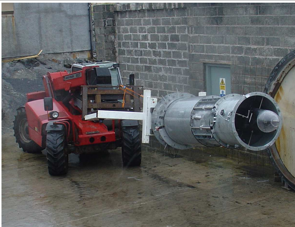
Figure 9: Installation of prototype Wells turbo generation unit at LIMPET on Islay
