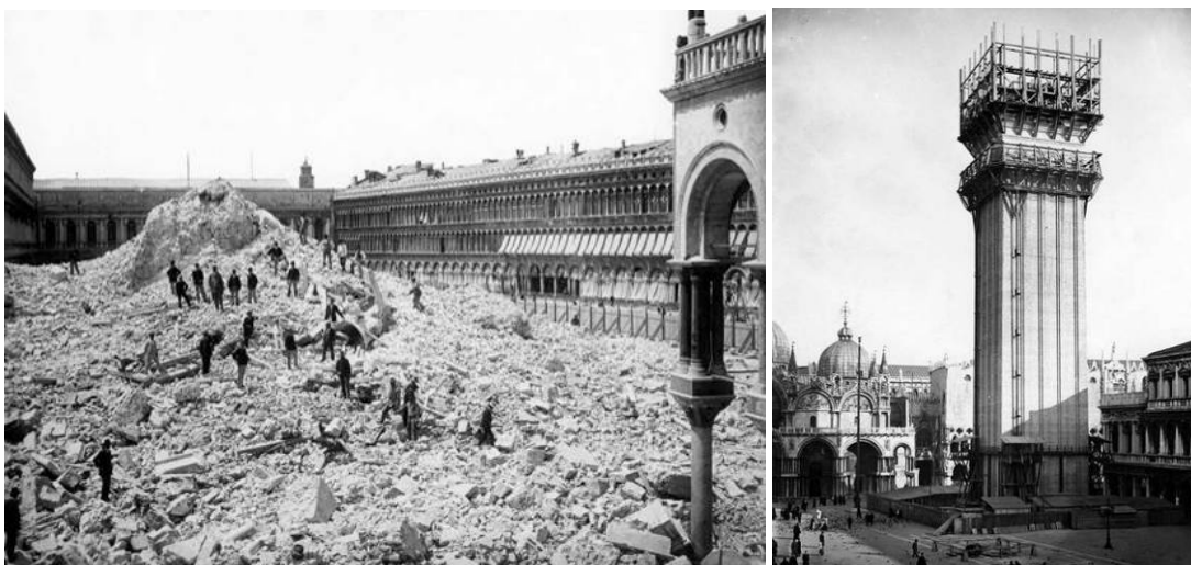
Figure 30. Campanilla di San Marco, Venice collapsed in 1902 and was reconstructed as an exact replica over the next ten years.
