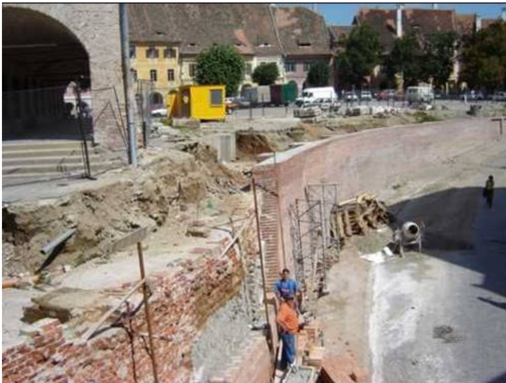
Figure 112. Sibiu, Lies' Bridge under restoration.
