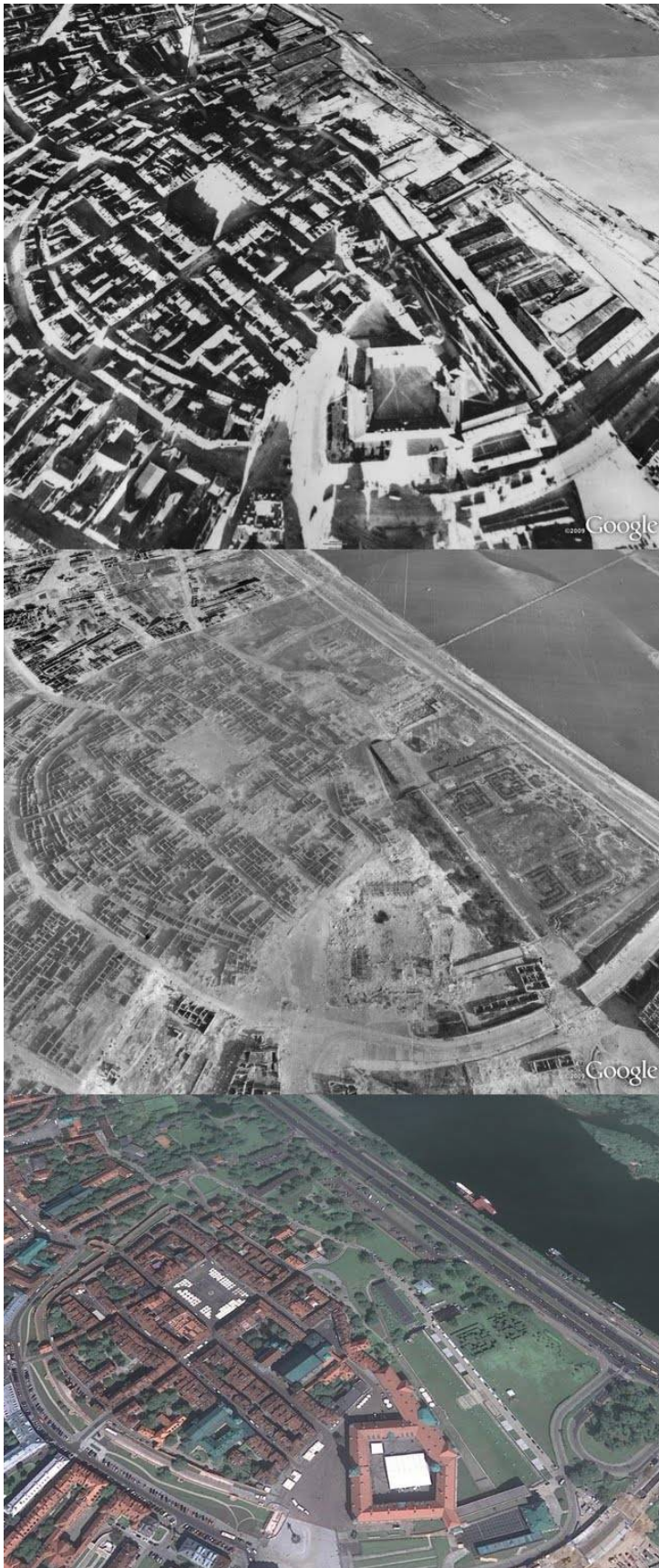
Figure 24. Aerial views of Warsaw Old Town in 1935, during the reconstruction in 1945, and now
