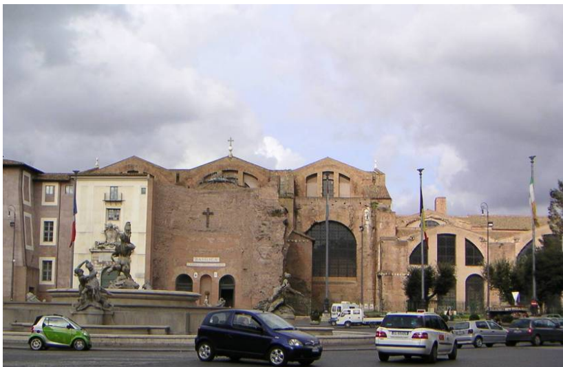
Figure 76. Entrance of Santa Maria degli Angeli e dei Martiri (Michelangelo, 1561 with façade after the 1911 restoration, stripped of the Neoclassical layer added by Luigi Vanvitteli, 1748-65)
