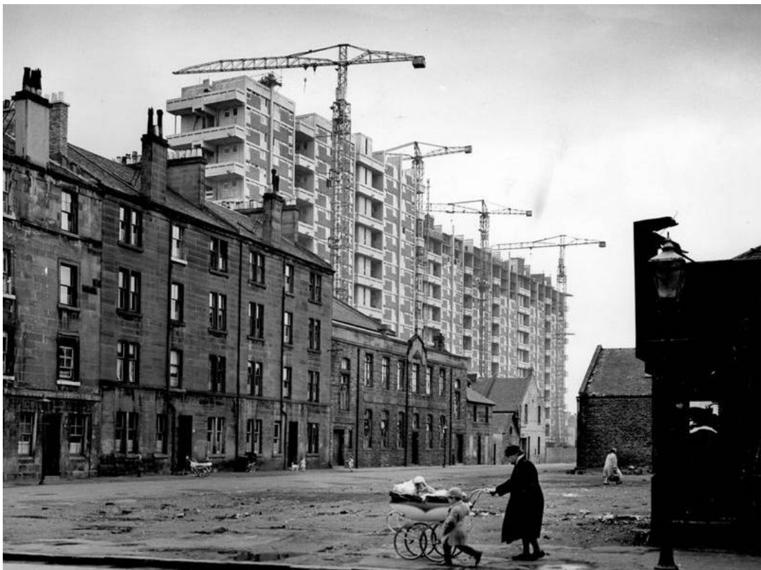
Figure 31. In 1960s, Basil Spence's tower blocks replaced old tenements in Glasgow's Gorbals
