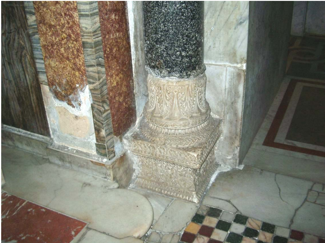
Figure 43. S. Prassede, Rome, capital re-carved into a column base and slices of ancient marble columns re-used as wall facing and floor mosaics
