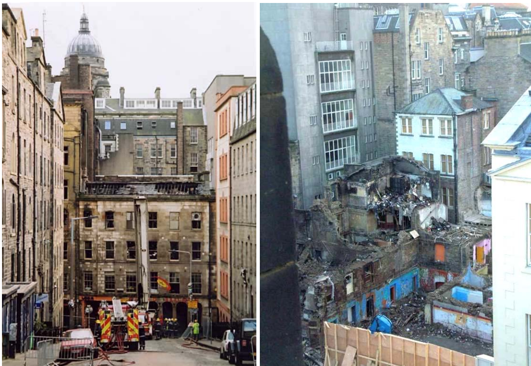
Figure 99. Edinburgh 2002 fire site in Cowgate before and after the demolition of the façades
