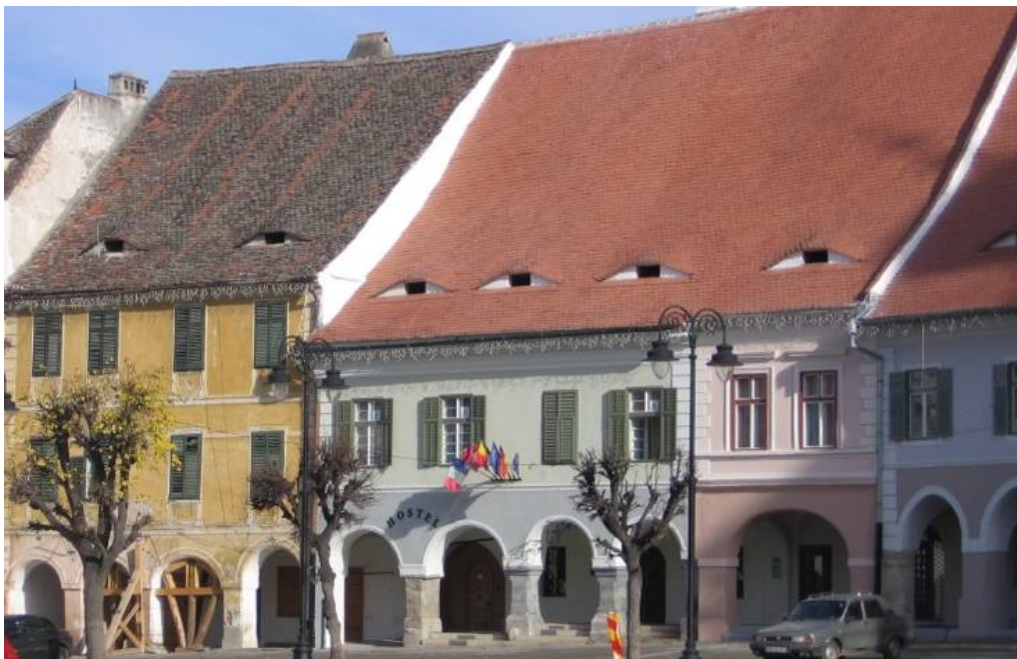
Figure 135. Sibiu roofs' 'eyes' are placed under protection
