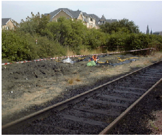
Figure 1: Ballast contamination clearly visible adjacent to contaminated land
