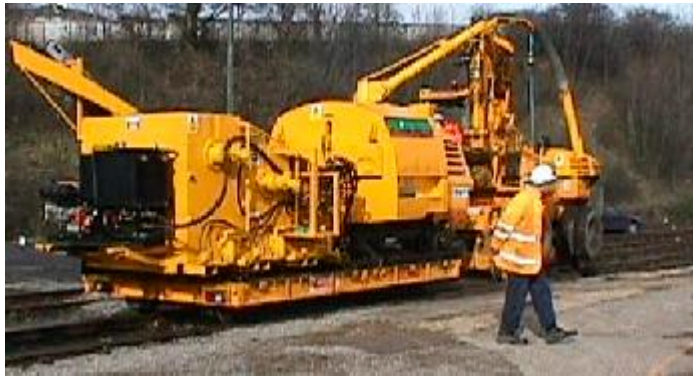
Figure 2: Track mounted ballast cleaning machine employing solvent washing
