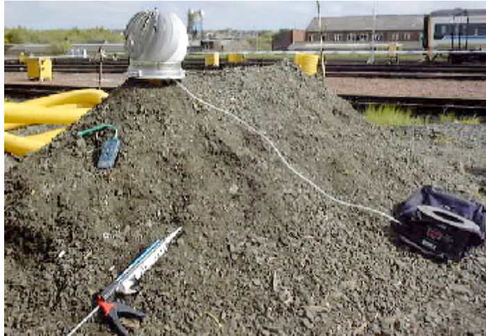
Figure 8: Biopile with vertical aeration pipes and aspirating cowl
