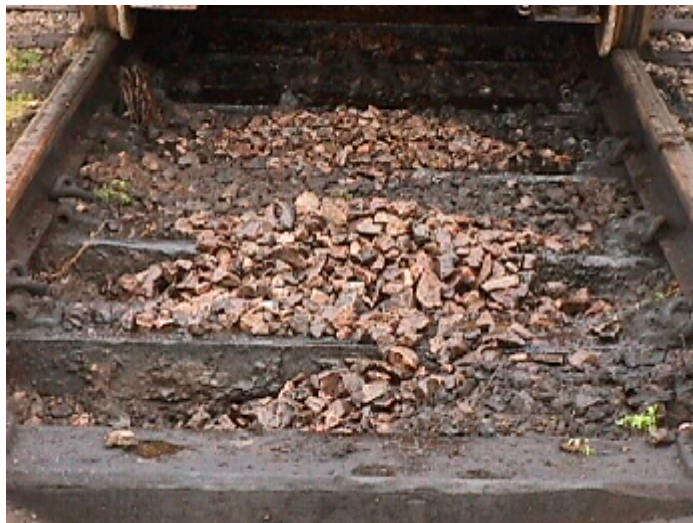
Figure 3: Cleaned ballast returned to the track
