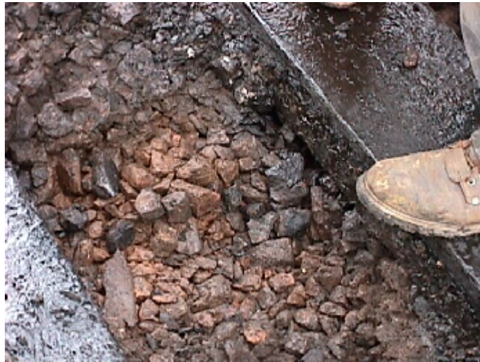
Figure 5: Extent of ballast removed by vacuum lifting
