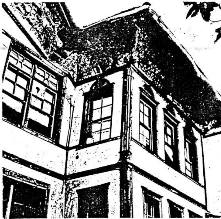
Fig.17 Many large openings on the upper floors towards the streets, (Moutsopoulos,1967, illustr.part,p.118).
