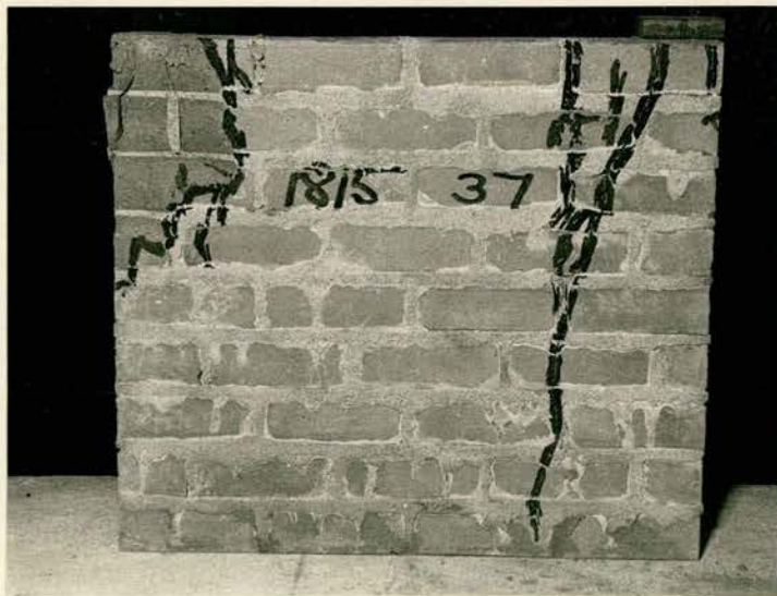
1/3rd. Scale Brick Wall - End Bearing Plate - Failures by Local Spalling, Crushing and Diagonal Cracking.
