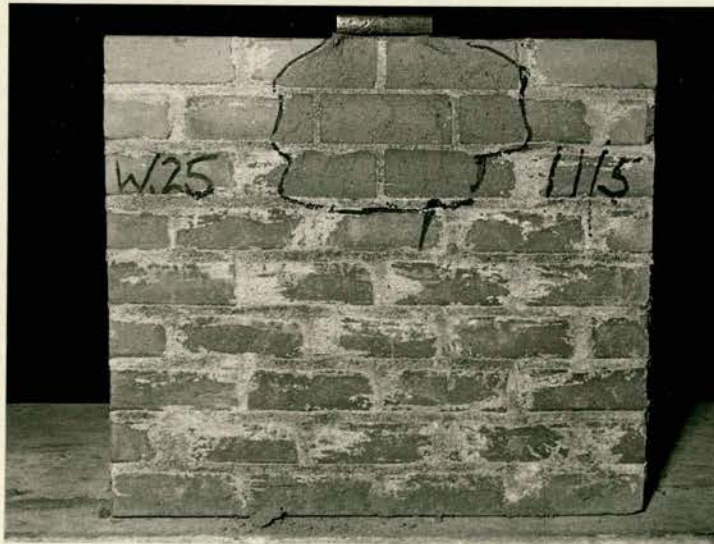
1/3rd. Scale Brick Wall - Central Bearing Plate - Failure by Spalling on One Face Only. Plate 6 - 10
