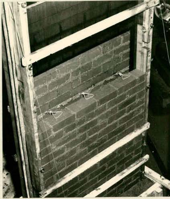
A Typical Stage in the 1/3rd. Scale Cavity Wall Construction.
