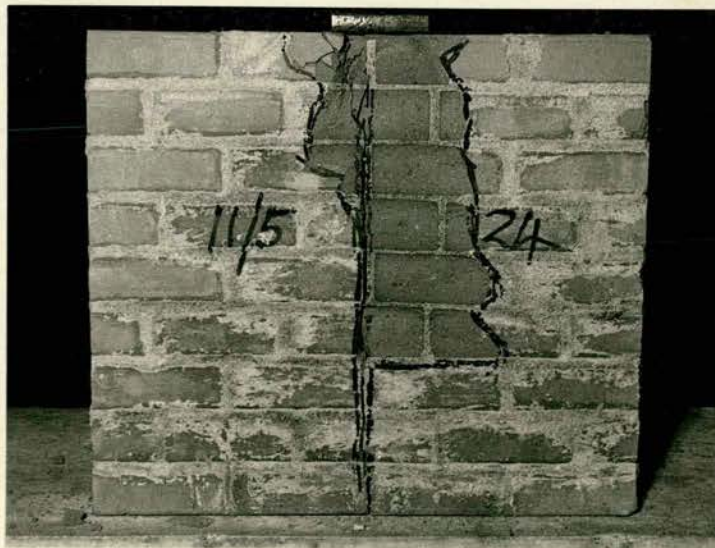
1/3rd. Scale Brick Wall - Central Bearing Plate - Failure by Vertical Cracking and Substantial Spalling. Plate 6-6
