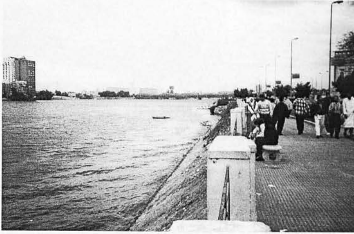
Figure 4.14: Example of walkways along breakwaters on the northern waterfront.
