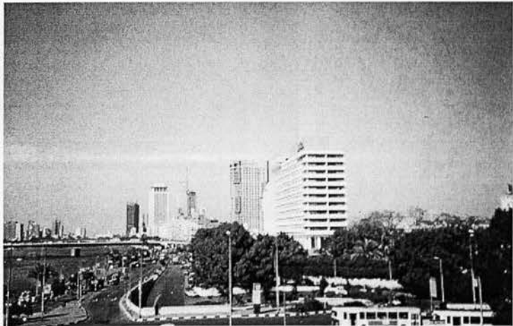
Figure 4.6: Hotels and office buildings occupying central areas of the Cairene waterfront.
