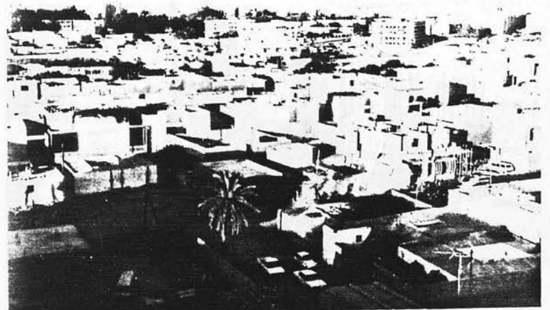
Fig 6.79 Steps have not been taken to ensure that this area is properly finished. There is no control of building nor any care taken of space between houses.
