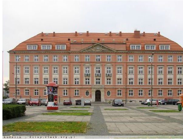
Fig. 30 Oberprasidium building after the restoration (source: dolny-slask.org)
