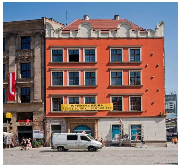
Fig. 12 Main Market Square Haus zur Goldenen Krone after the reconstruction modern picture (source: dolny-slask.org.pl)
