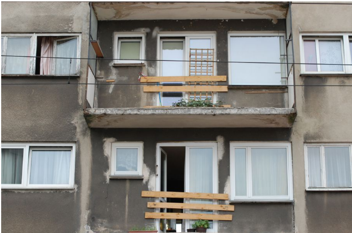
Fig. 22 Provisionally secured balconies on eastern side of the square (author's own)
