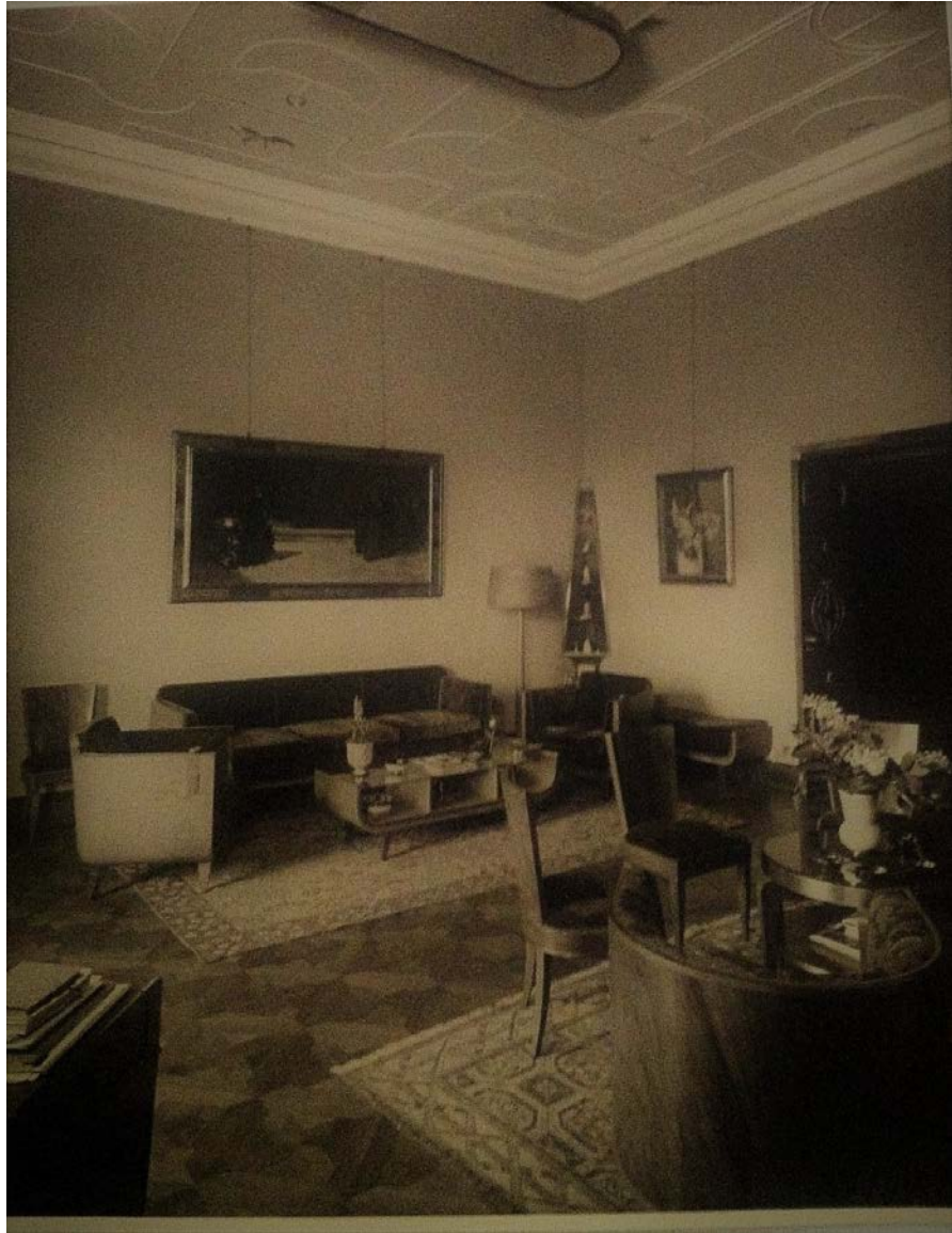
Figure 13. Photograph of Villa Vittoria, Florence, Interior.
