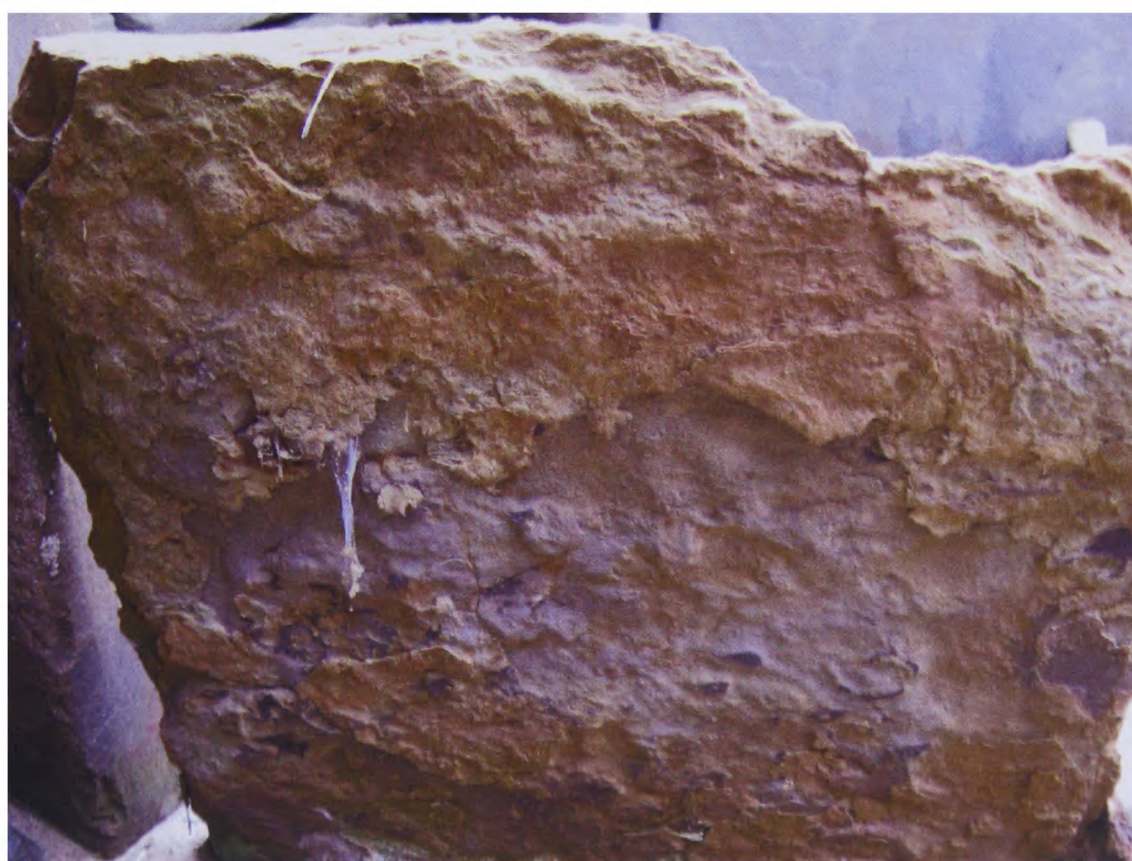
Figure 5.6: Another area showing dramatic decay. Photograph taken during the March (2004) visit. Stone slab is approximately 57 cm high, 52 cm wide and 3.5 cm thick. Area 4.
