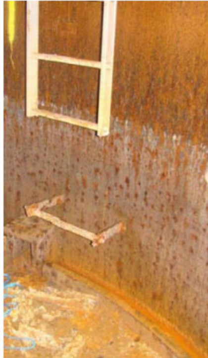
Figure 2.5: The lower part of an aluminium ladder above the lower working platform has corroded away due to tidal conditions inside an offshore wind monopile foundation [14].
