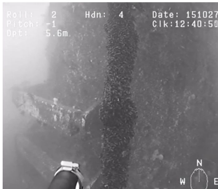
Figure 6.14: Clusters of Blue mussels by the anode cage at 5.6m depth on WTG A08.
