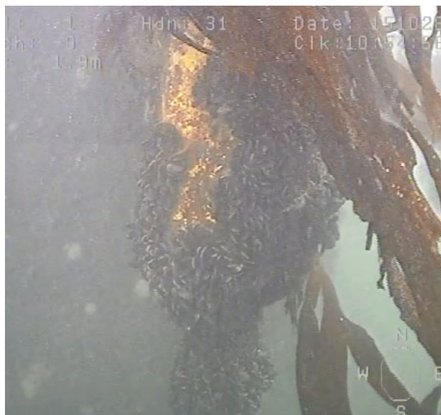
Figure 6.13: Kelp/Blue mussel transition zone at 1.9m depth on WTG B17.
