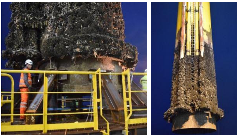
Figure 2.9: Decommissioned TP from Robin Rigg Offshore Wind Farm.
