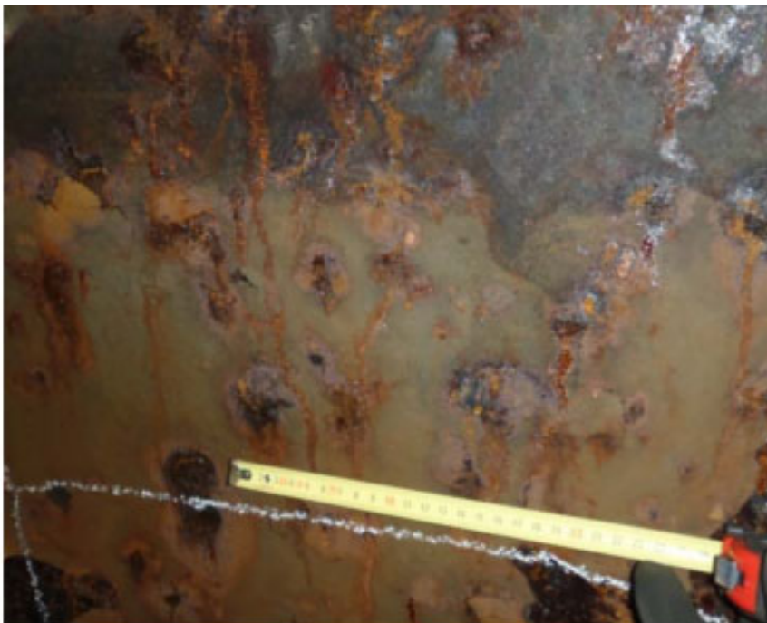
Figure 2.5: The lower part of an aluminium ladder above the lower working platform has corroded away due to tidal conditions inside an offshore wind monopile foundation [14].
