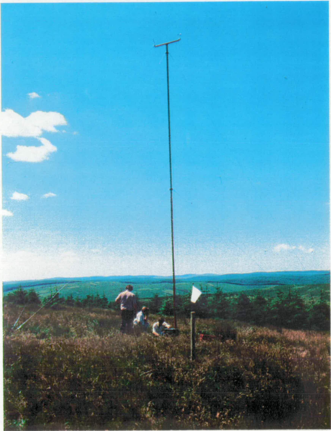
Figure 3.1 Photograph of wind measuring equipment installed at Cwm Berwyn, a hill top site in mid Wales. View south-westwards on an exceptionally calm day, with the monitoring forest visible on the hilltop in the middle distance.
