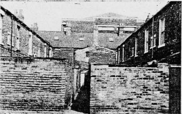
The terraced housing is cramped front and rear, the houses themselves small, without inside lavatories or bathrooms.
