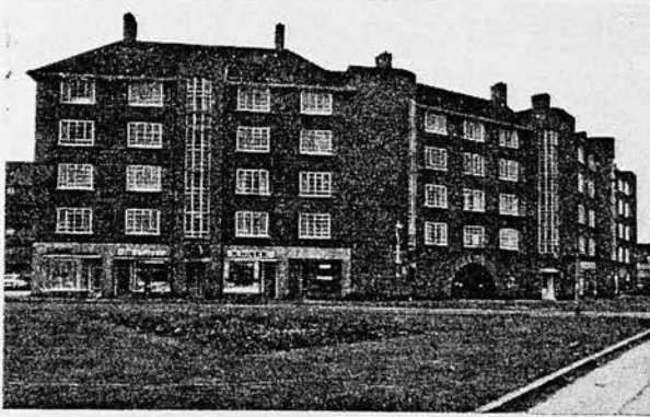
1930's council flats — the result of inner city slum clearance.
