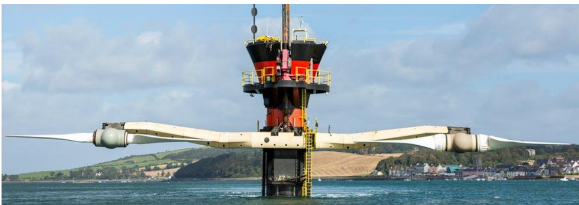
Figure 2-8: 1.2MW MCT SeaGen installed in the Strangford Loch, Northern Ireland. Image copyright of Sea Generation Ltd sourced: www.seageneration.co.uk .
