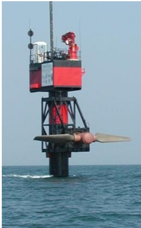
Figure 2-7: 300kW MCT Seaflow installed in 2003 off Lynmouth, Devon. Image copyright of Marine Current Turbines Ltd, sourced: www.british-hydro.org .
