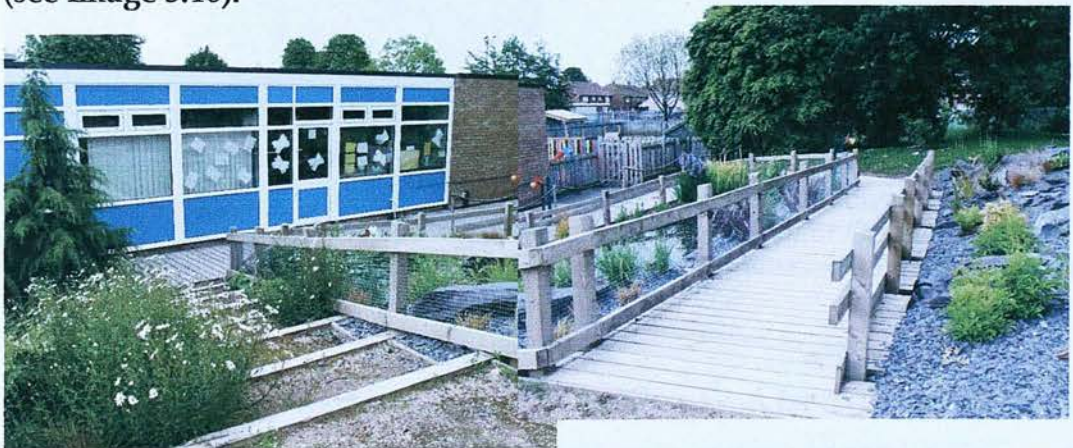
Image 5.16: Some users preferred using the steps instead of the ramp at the end of the boardwalk, even though they were in their wheelchairs, due to the slippery surface.
