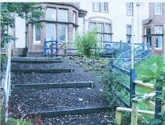
Image 1.7: Steps like this are common in a sensory garden. As a result, wheelchair users are not able to access some parts of the garden.
