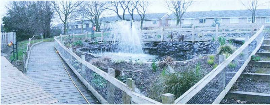
Image 1.8: This ramp is hardly used due to its slippery surface, especially when damp, while the stairs are inaccessible to wheelchair users. Consequently, users use another route for access.
