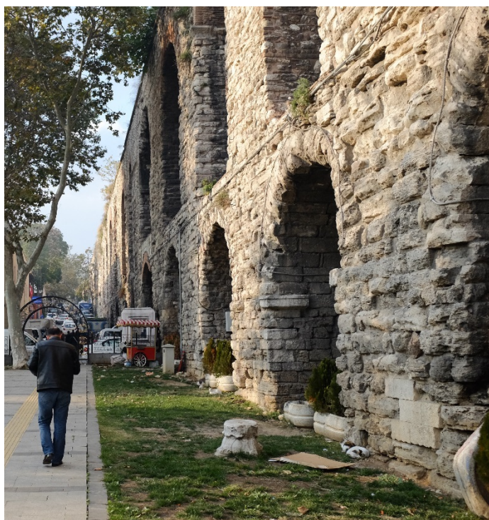
Figure 2.1: The 1km-long Bozdoğan Kemerleri: almost all of it remains today. Carrying water across the deep valley between Hill Four and Hill Three, it is the most visible part of the city's ancient water supply. (Photo: S. Smith 2014)
