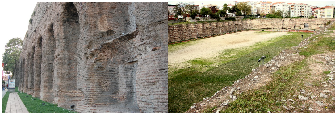
Figure 3.2: The Unkapanı and Fildamı cisterns. Left – exposed wall of the Unkapanı cistern with buttress style construction, the rear of the cistern is embedded in the hill. Right – the Fildamı cistern with the exposed front wall in the foreground and in the background the buttressed back wall which supports the ground behind.
