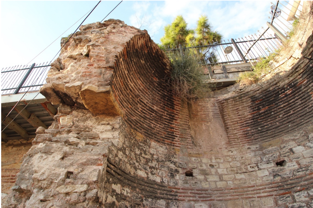
Figure 6.12: The remains of the Aspar internal tower showing an opening (left) and the blocked up opening in the dome (centre) photo: K Ward.
