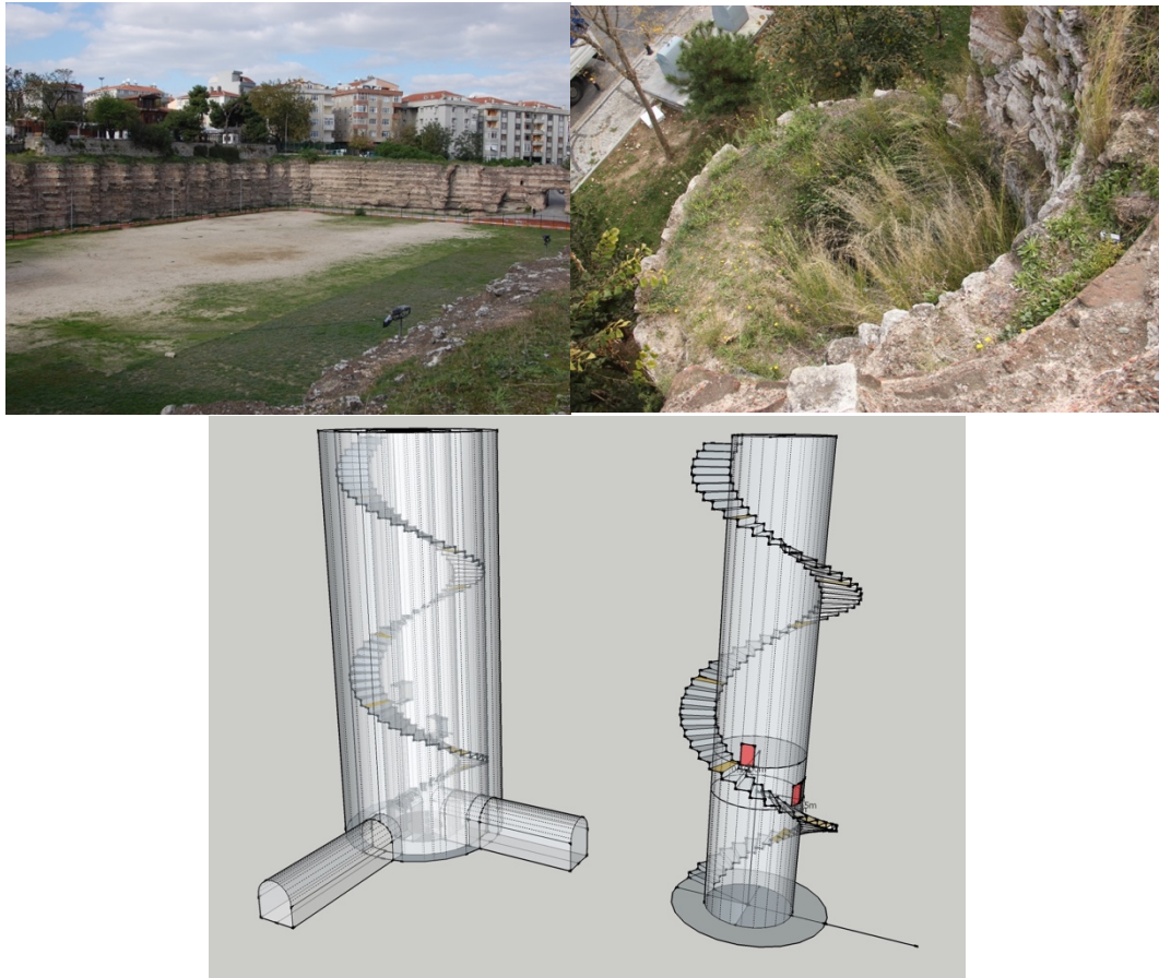
Figure 6.13: Fildamı cistern details. Cistern interior (left). Remains of control tower from above (right) and sketch (F Ruggeri) of the Fildamı tower.
