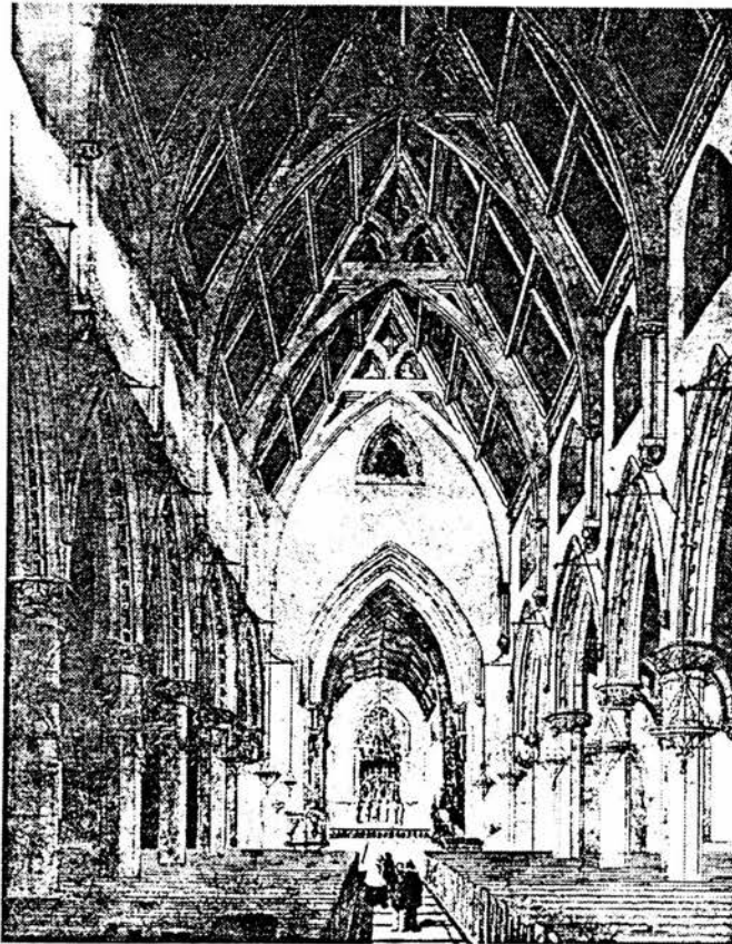
Fig.112 Interior of Christ Church Cathedral
