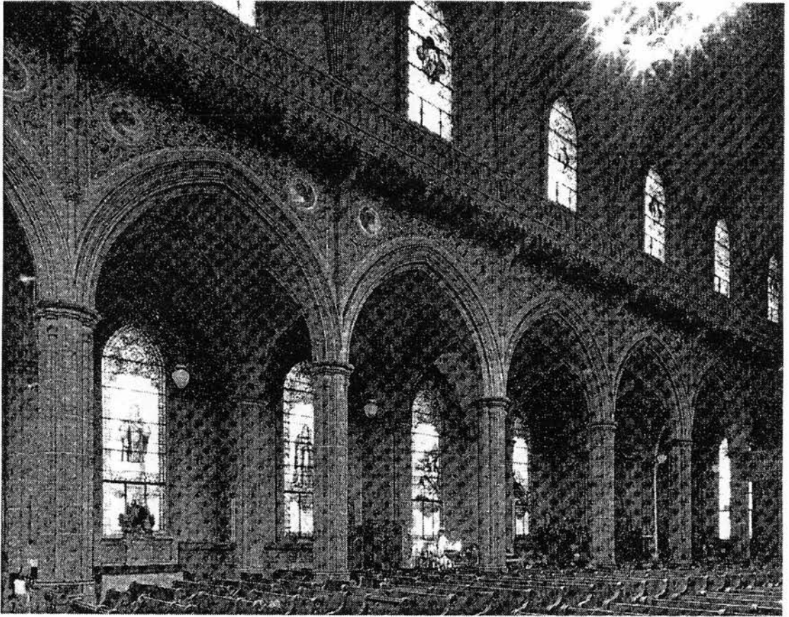
Fig.101 View of clerestory and aisle, Church of St. Pierre Apôtre
