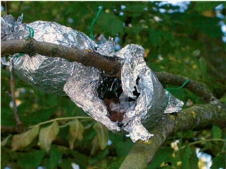
Plate 24 : Serious damage on air-layered branch.
