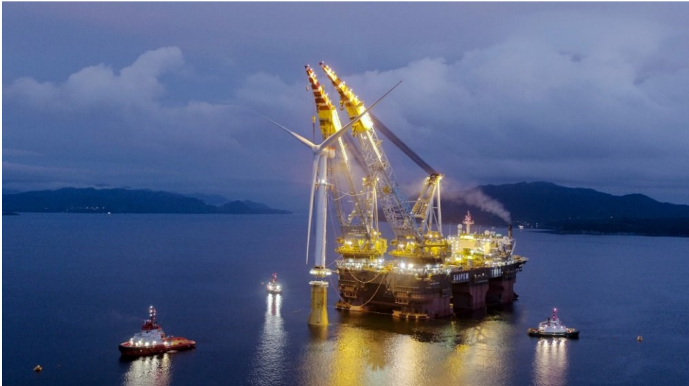
Figure 1.1. A 6.0 MW floating wind turbine with a rotor diameter of 154 m being installed in 2017 as part of the 30 MW Hywind Scotland project (Equinor, 2018).
