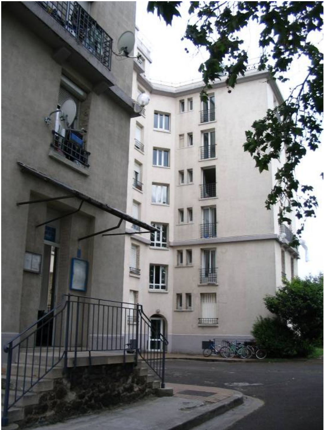
Figure 2. At the entry to the building (#2)
