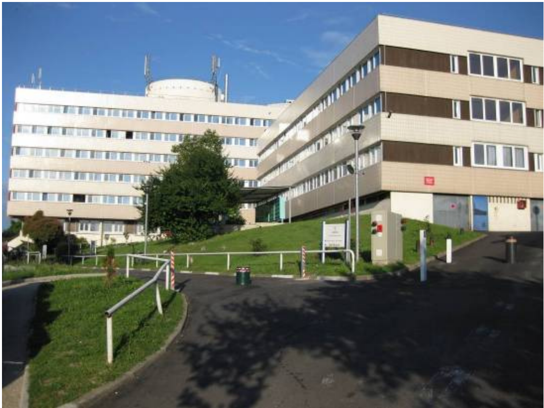
Figure 1. At the entry to the building
