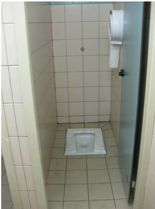
Figure 9. Shower block and squat toilet.
