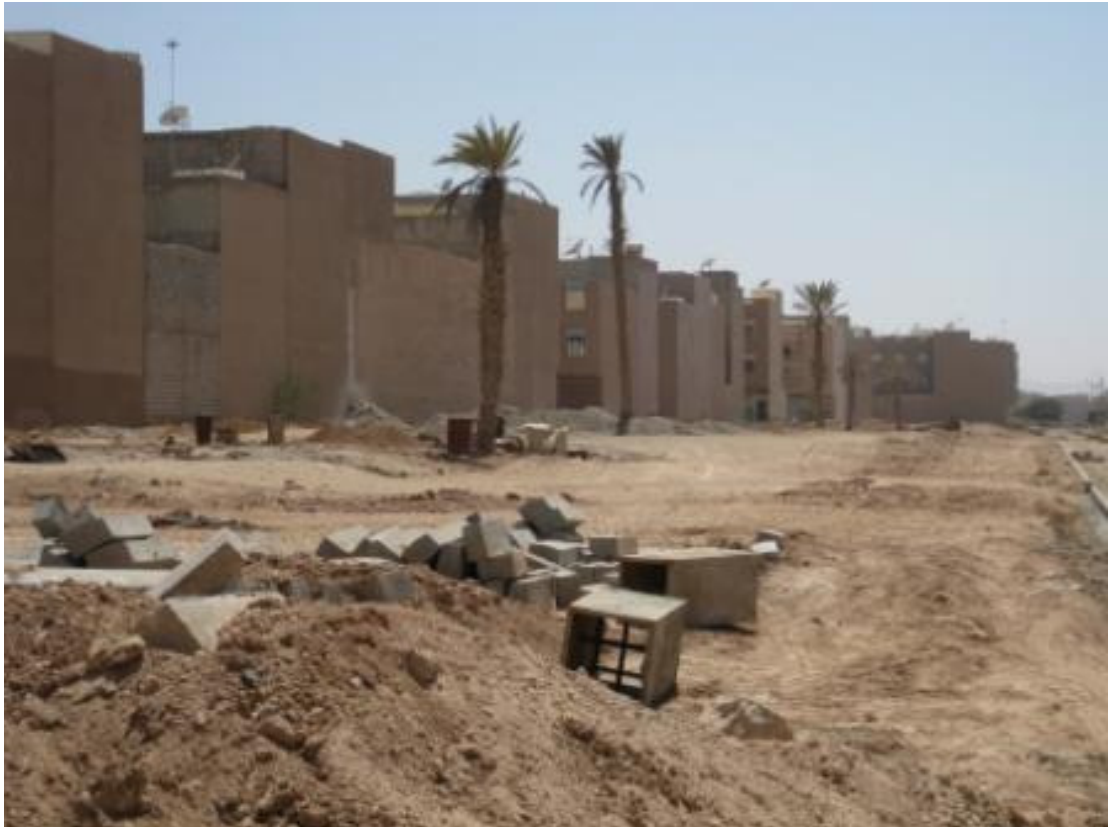
Figure 28. A new housing development under construction on the outskirts of Tiznit.
