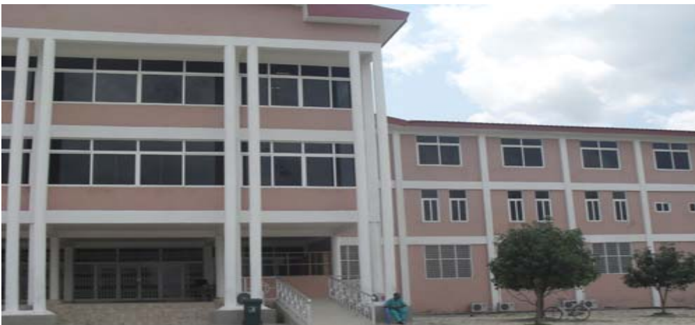
Bolgatanga Polytechnic: Library Complex
