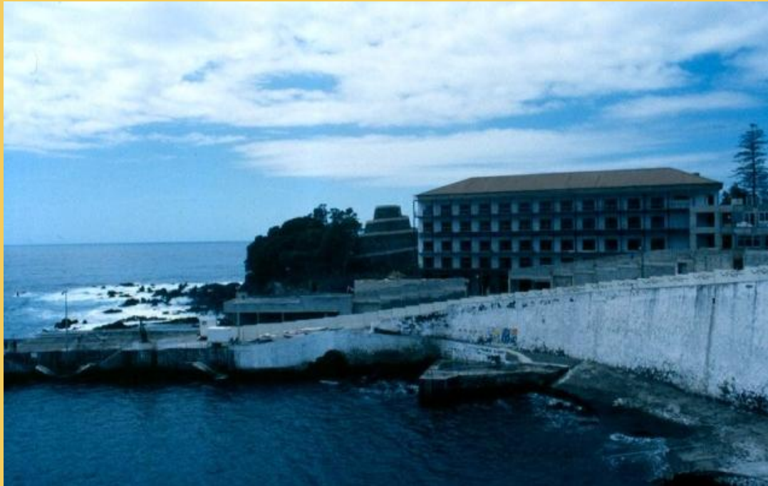
Figure 15.4 Construction of hotels in the surroundings of the property of Angra do Heroísmo
