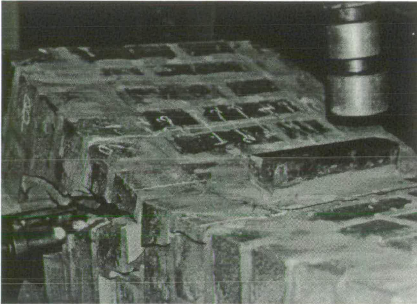
Fig 4.5-38 : A typical diagonal shear failure within the shear span
