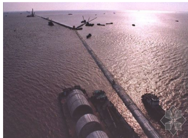
(b) Installation of the standard caisson on a mound structure
