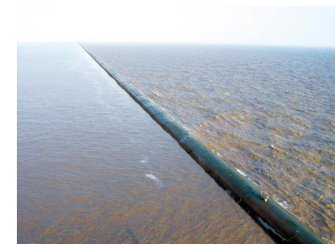
(c) Completion of construction project
