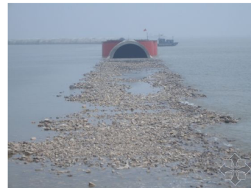
(b) Installation of the standard caisson on a mound structure
