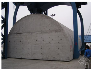
(a) Handling of the semicircular caisson unit
