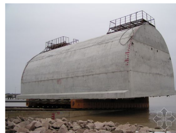
(a) Handling of the semicircular caisson unit
