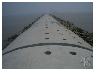
(b) Installation of the standard caisson on a mound structure
