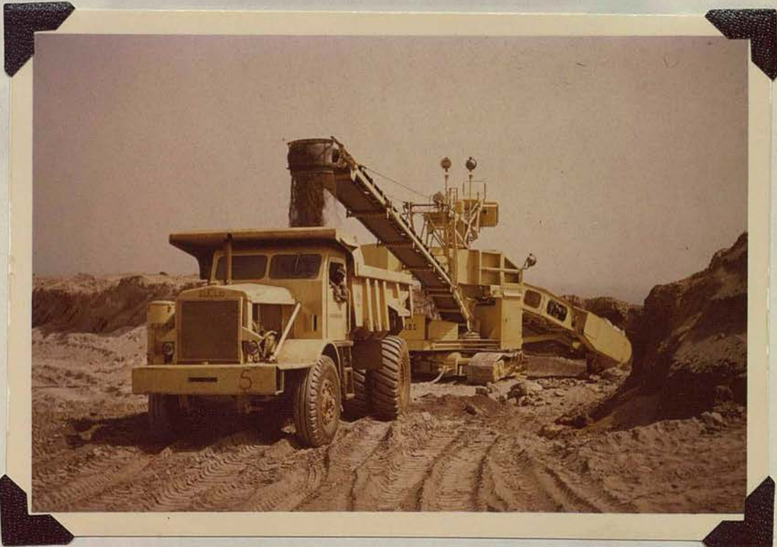
14. Removal of overburden. S.L.D.C. Marampa.
