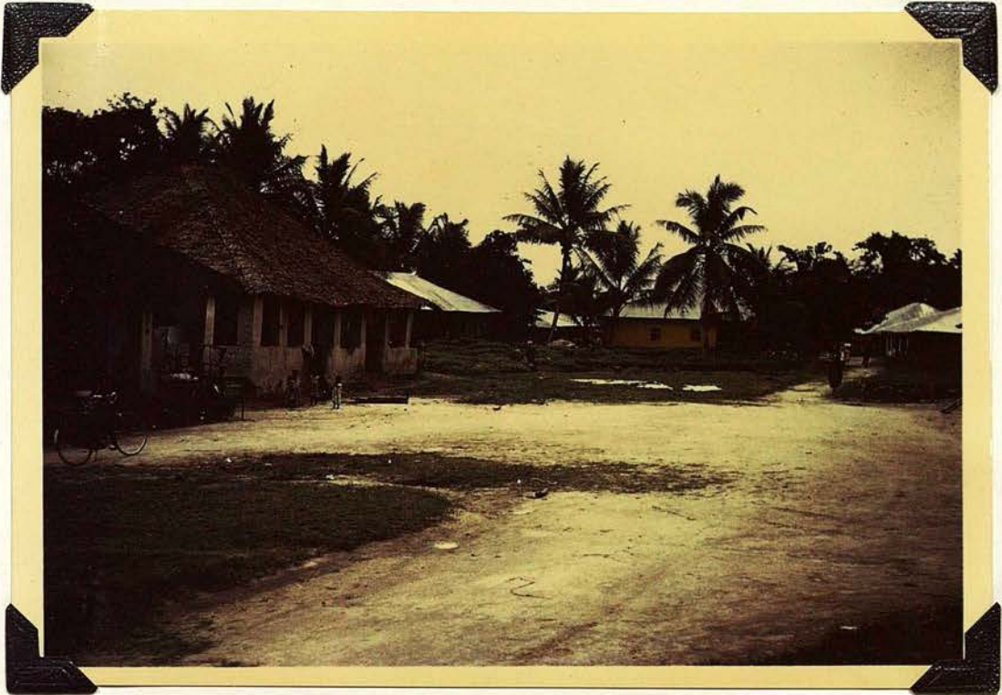
3. Old Lunsar. Note construction of houses.
