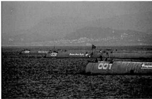
(a) World's first wave farm, Aguçadoura, 5km north of Porto, Portugal comprising three Pelamis P1 750kW devices.
