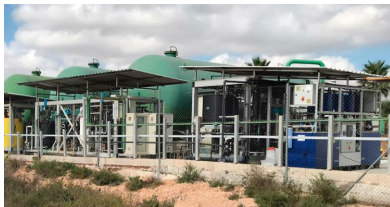
Figure 29. Reverse osmosis desalination solution that allows the recovery of phosphorus. (Retema, 2021)
