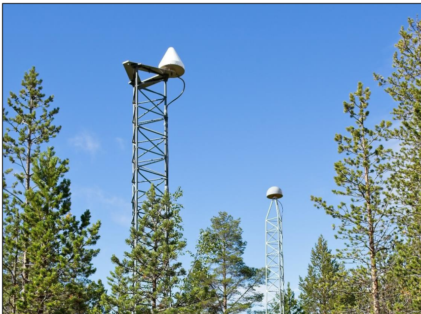
Figure 10. Old antenna mast (front) and new mast (behind) at the dual station Kevo. The old mast had a triangle shaped platform that caused multipath and the radome was conical. In the new construction the top of the mast is narrowed and the radome is spherical. Photo J. Näränen.
