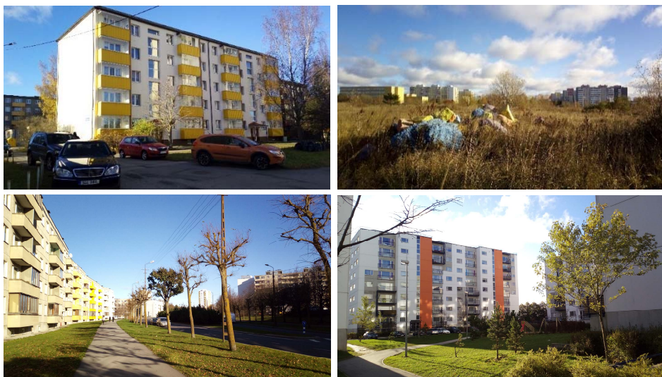
Figure 1. Top left: refurbished building in Mustamäe; bottom left: a view of the housing placed in a circular fashion in Väike-Õismäe; top right: a view of undeveloped municipal land in Lasnamäe; bottom right: Raasiku housing development in Lasnamäe. Source: Author's photographs.
