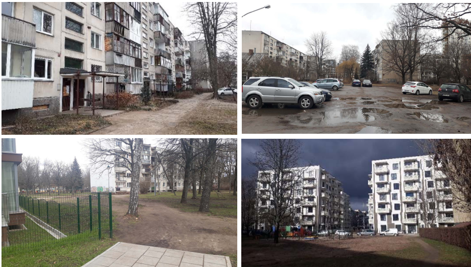
Figure 3. Views in the Žirmūnai triangle. Top left: typical local housing; top right: parking problems in the area; bottom left and right: on both pictures we can see the gating of new infills and how development occurs only within the borders, not taking into account the adjacent public areas. Source: Author's photographs.
