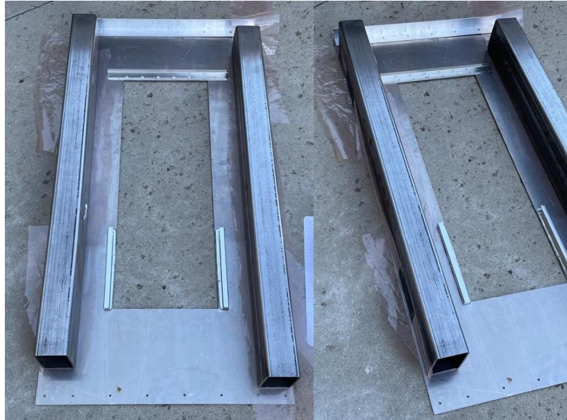
Figure 23: Shows the riveted portions of the door and the composite flanges being epoxied to the door.
