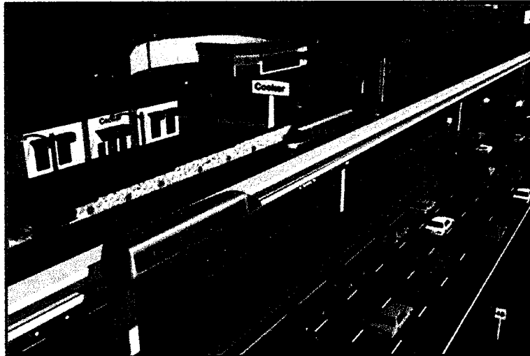
Figure 2.4: Transit cantilevered monorail (Kennedy, 2010).
