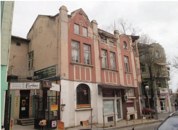
Fig. 9. Terrestrial photo from a person's point of view
