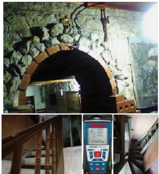
Fig. 12. Interior photos and Bosch measuring device
