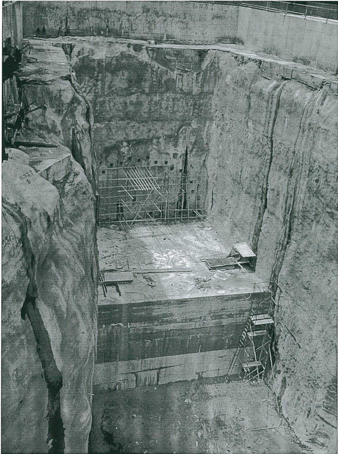
Figure 1 Foamed concrete application at the SMART tunnel in Kuala Lumpur
