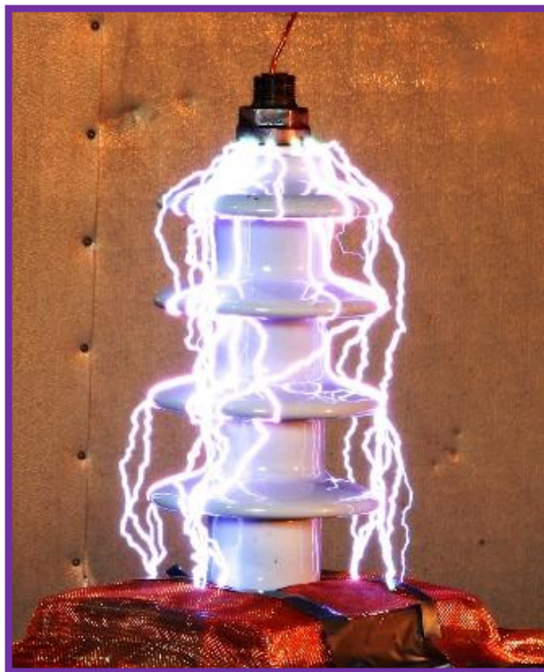
Figure 2.6 : Flashover occurred on surface of insulator [10]
