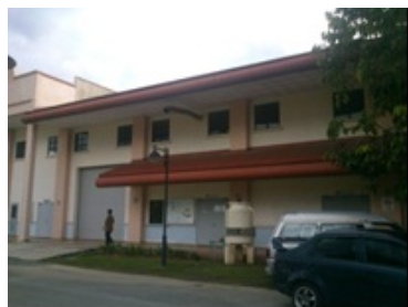
Fig. 3 Block E laboratory building
