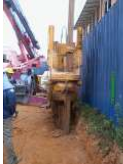
Fig. 2.1: The sheet pile installation at Bukit Serdang, Malaysia (2014)
