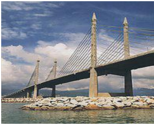
Figure 1: Penang Bridge, Malaysia
