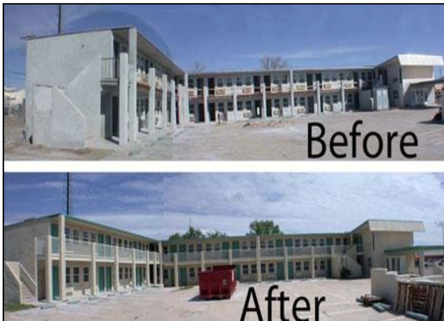
Figure 3.3: Pictures showing the Refurbishment and Fit-out
