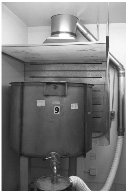
Figure 2.8: Large mixing ventilated booth-type exhaust hood (Old et al., 2008)
