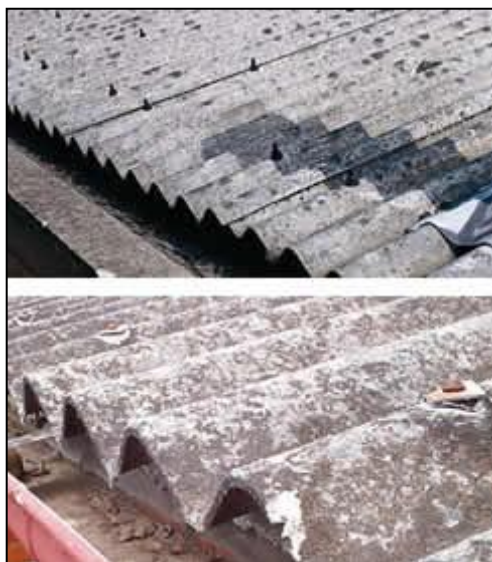
Figure 2.4 : Asbestos cement-roof (Chiesa, 2010)
