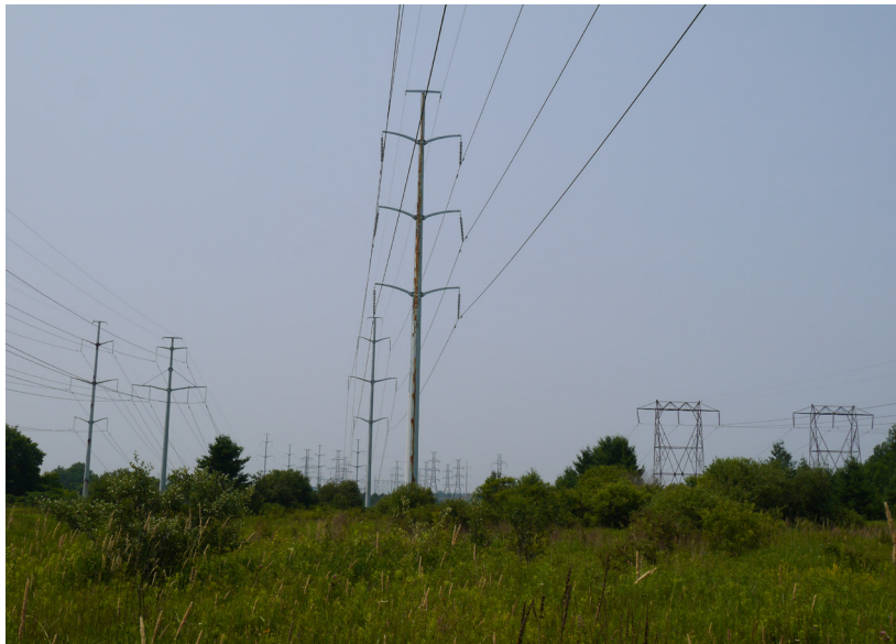
Figure 21: Some of the powerlines in the park, in the low vegetation underneath birds are found. For safety the ground underneath the power poles have bare to low vegetation.
