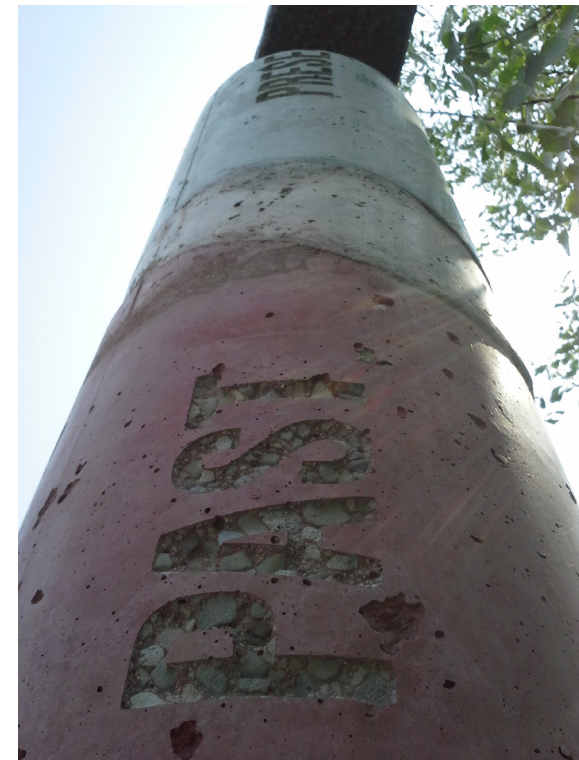
Figure 64: Pole at Evergreen Brickworks.
