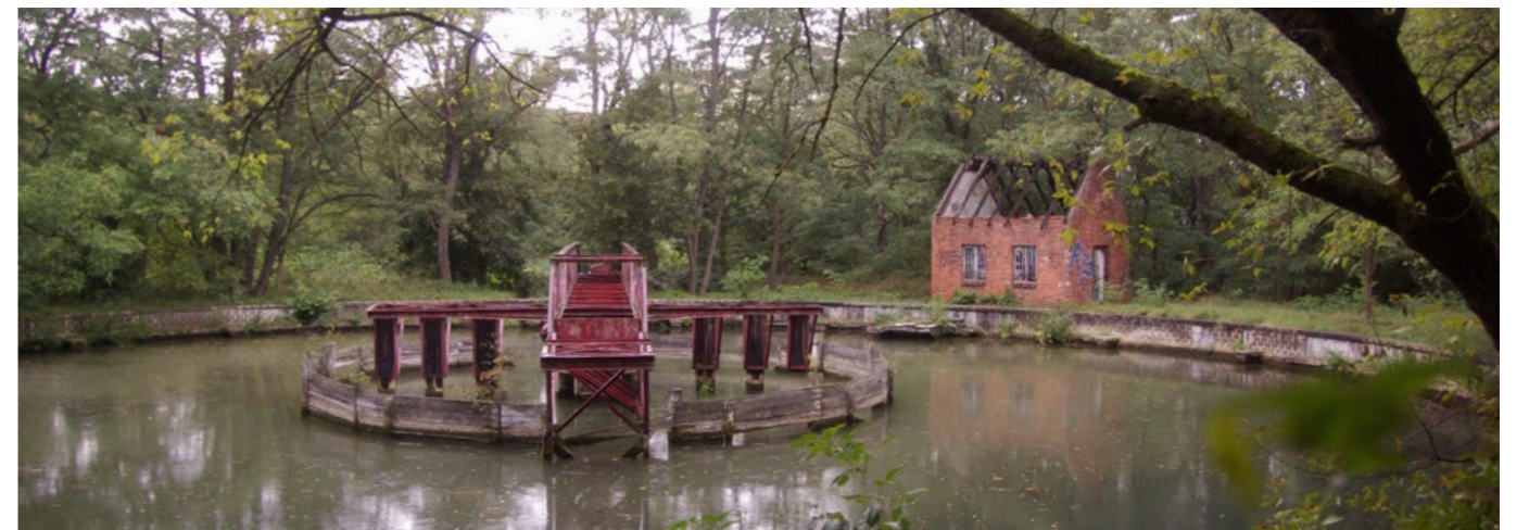
Remnants of the Treatment Plant.
