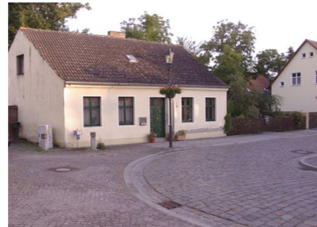
The east corner.
